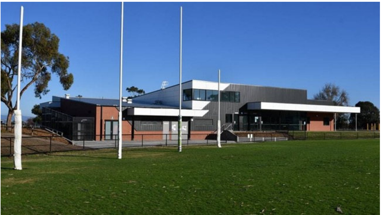
Figure 13: New Multi-Purpose Facility
