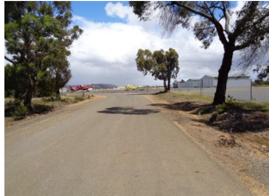
Access road/boundary fence looking south
