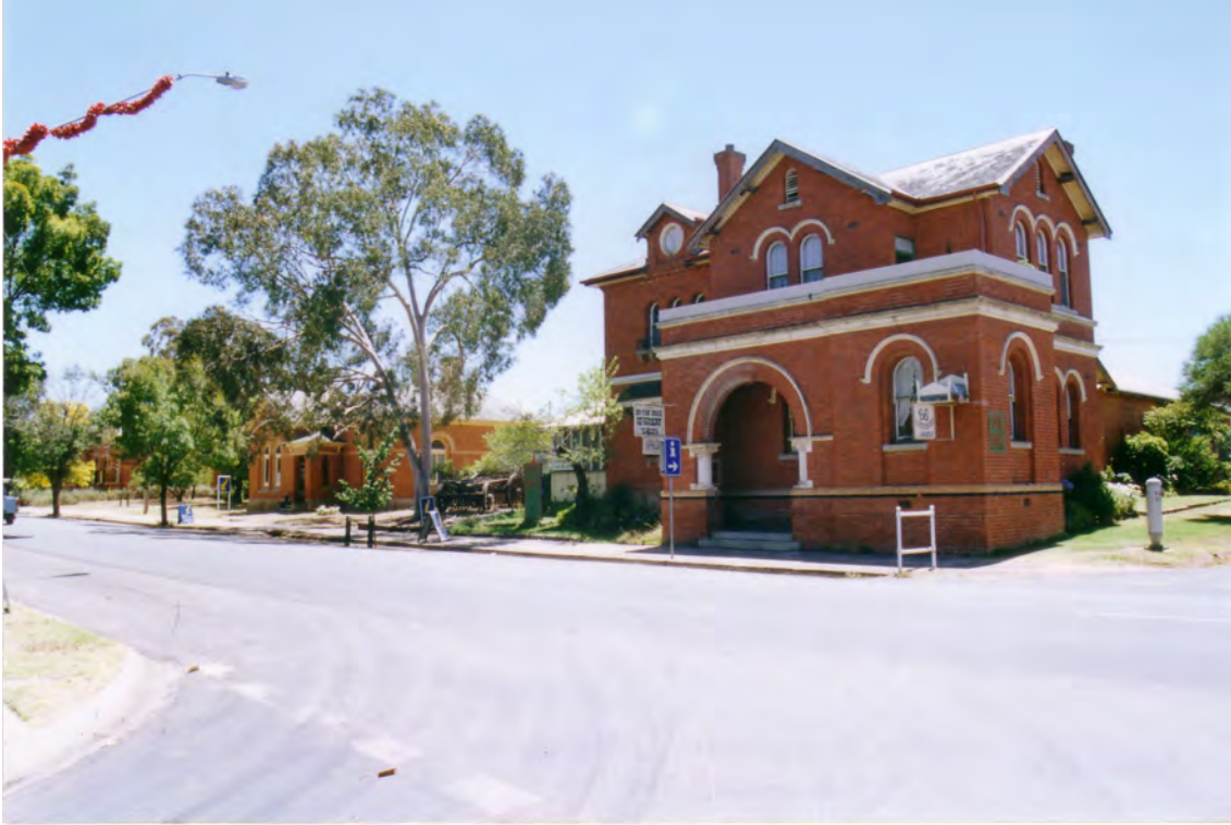
Photo 3.01: The Former Post Office, Land Office and part of the former Kara Kara Shire Offices in the background, Napier Street.
