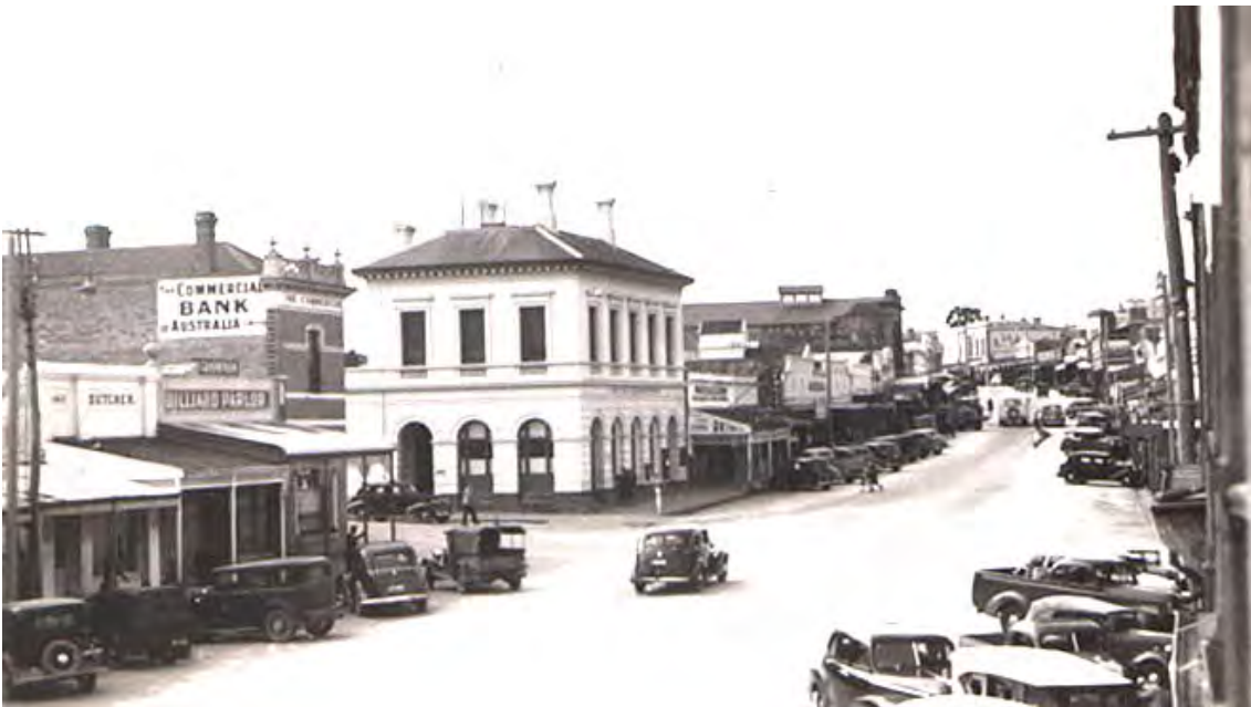
Figure 8.10: Main Street, Stawell, c.1935. Source: Stawell Historical Society (D05c_SHS_0366a)
