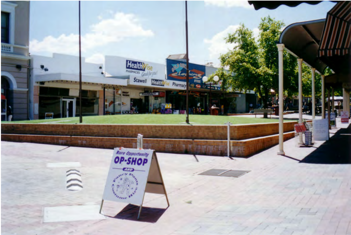
Photo 8.05: Main Street showing new and substantially altered buildings with new shopfronts and overly proportioned parapets and projecting cantilevering canopies. Note the early roof monitors and gabled roof forms behind some of the introduced parapets.
