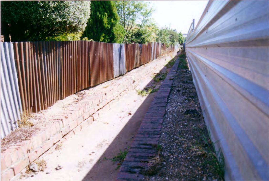
Photo 4.03: Brick channel in Queens Avenue, west side.
