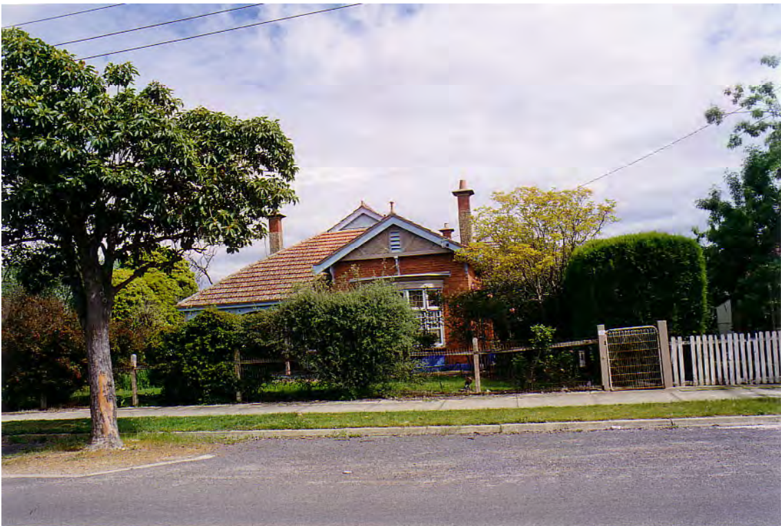
Photo 7.02: Example of a typical single storey, face brick Federation styled house in Skene Street with a hipped and gabled roof clad in terra cotta tiles. Also note the early timber post and woven wire fence.
