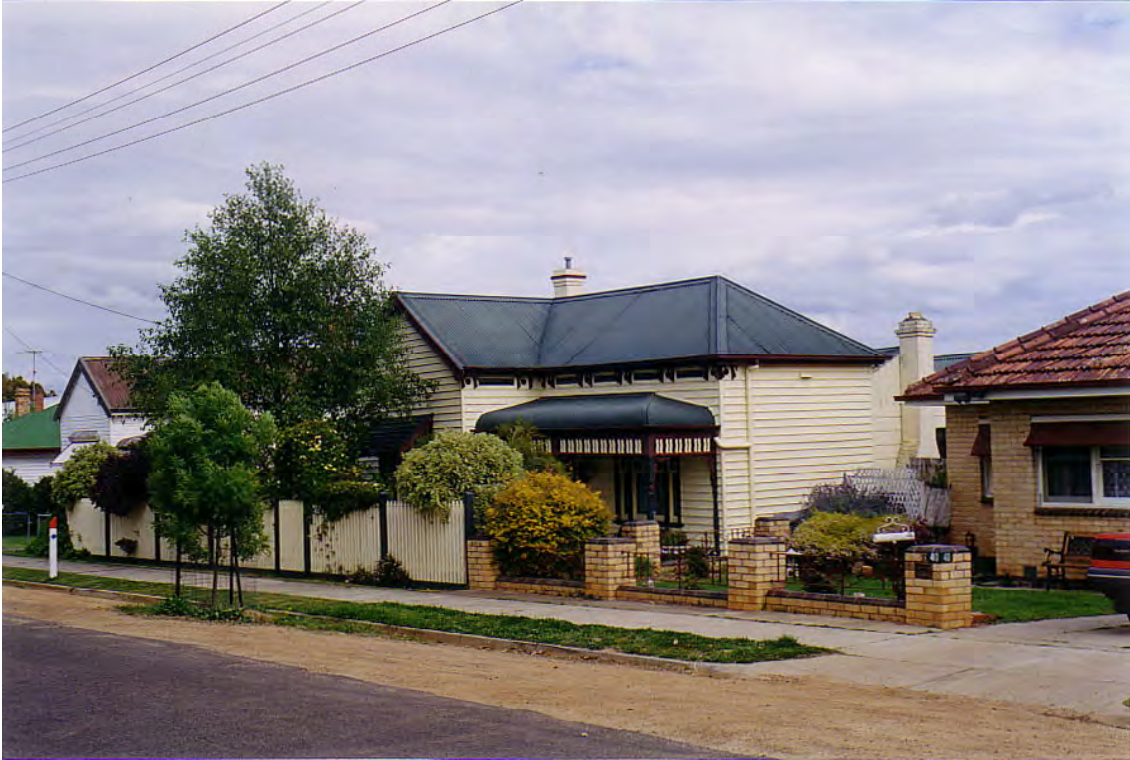
Photo 7.01: Example of a typical single storey, horizontal timber, weatherboard Late Victorian/Edwardian styled house in Skene Street with a hipped and gabled roof clad in galvanised corrugated iron.
