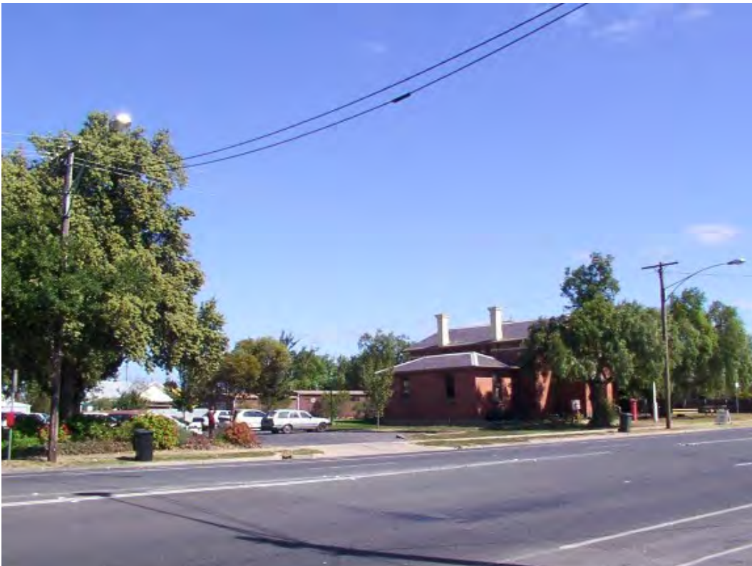
Photo 5.02: View of the former Court House, Longfield Street, Stawell. Also note the large side setback which now forms a car park.
