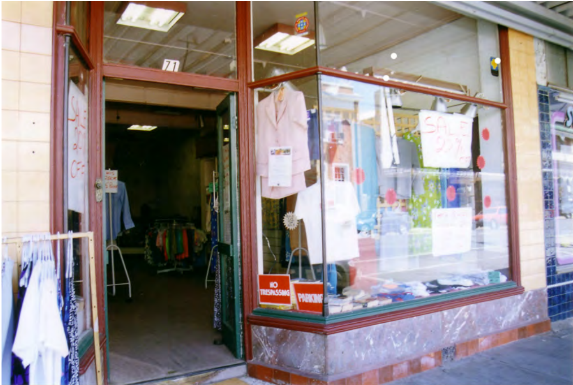
Photo 1.03: Shopfront with ingo detail, 71 Napier Street
