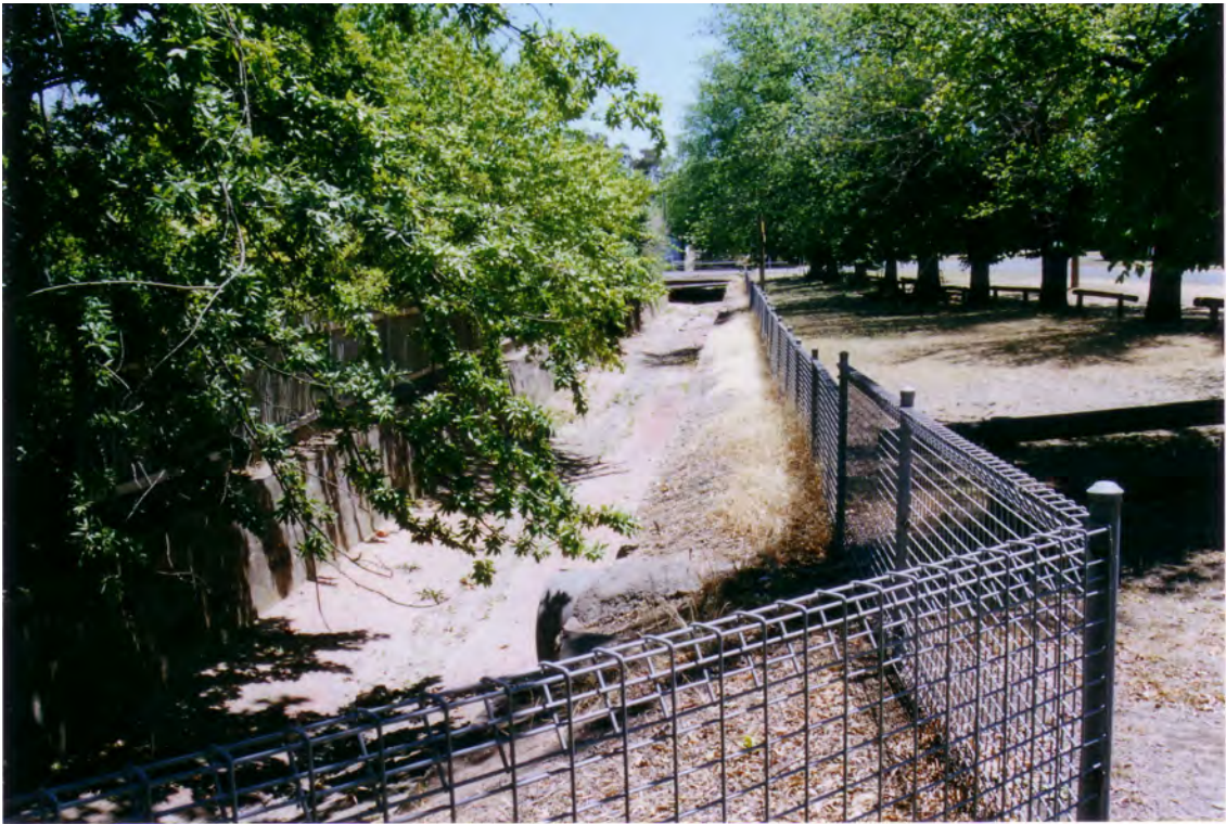
Photo 3.09: View of the early brick and stone drain on the west side of Napier Street
