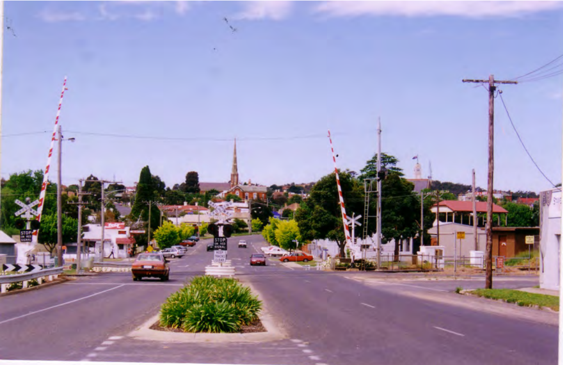
Photo 6.04: Seaby Street (north-east end), with views to the central Stawell township and the built landmarks including the spire of St Matthew's Church and the clock tower of the Town Hall.
