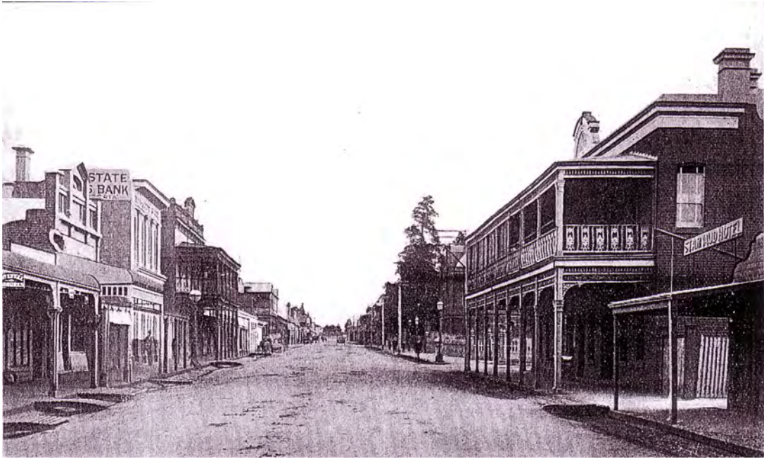
Figure 1.02: Napier Street. Looking north, [n.d] c early 20 th Century Source: Back to St Arnaud Souvenir of the occasion with Photographs of some of the Town's most interesting and picturesque features , Borough of St Arnaud Diamond Jubilee booklet, October 1921, p.7
