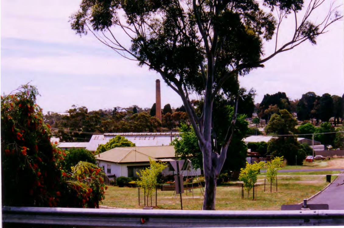
Photo 6.05: Seaby Street, with a view north-west to the chimney stack of the brickworks.
