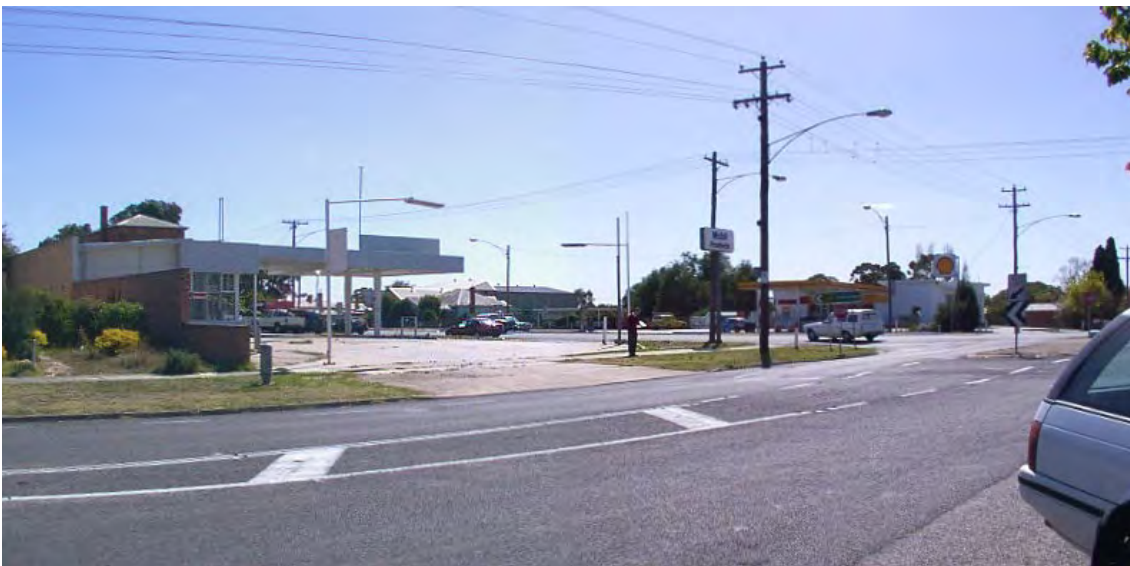
Photo 5.05: View of intrusive Service Station, corner of Longfield and Seaby Streets, Stawell.
