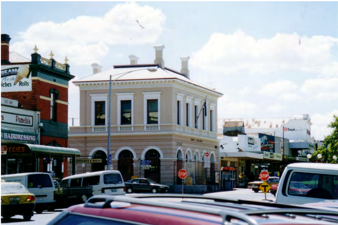
Photo8.0 8: View along Main Street showing introduced shopfronts and parapets, and the early gabled roof forms and monitor roofs (clad in galvanised corrugated iron) behind.
