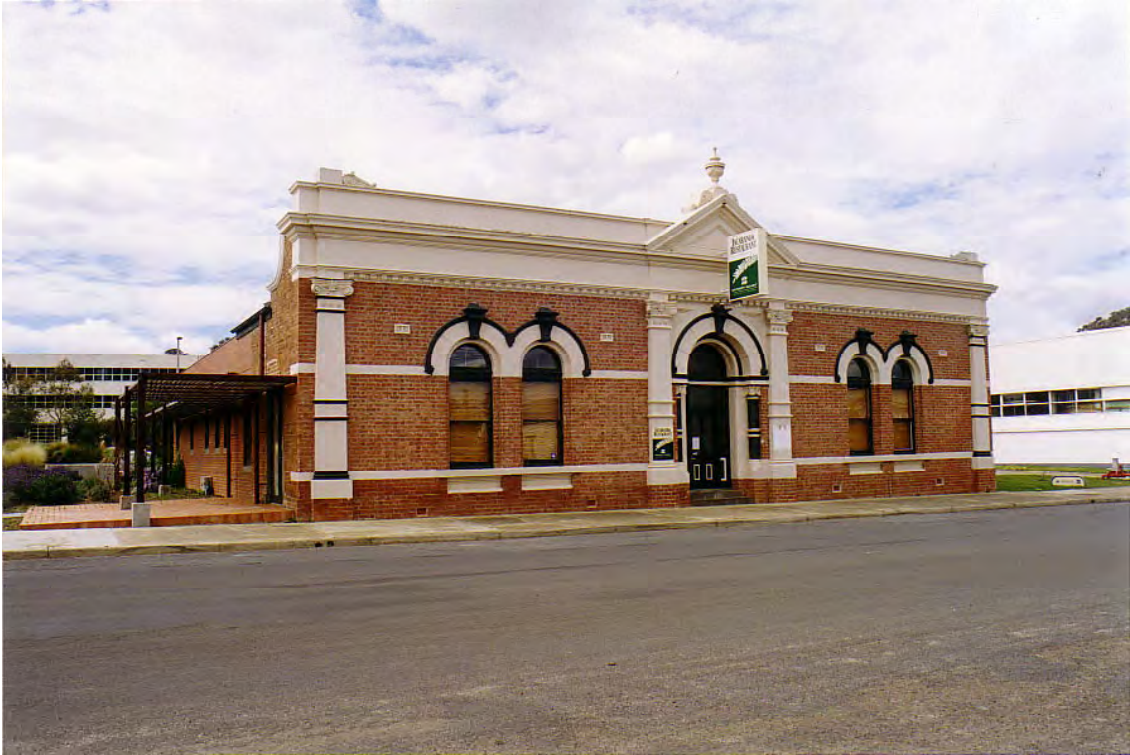
Photo 7.03: Former School of Mines Building, Skene Street.
