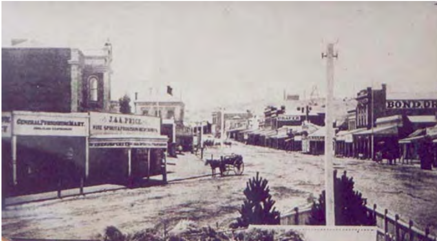
Figure 8.05: Lower Main Street, Stawell, c.1880. Source: Stawell Historical Society (Do2a_[c1880]_SHS_0537).
