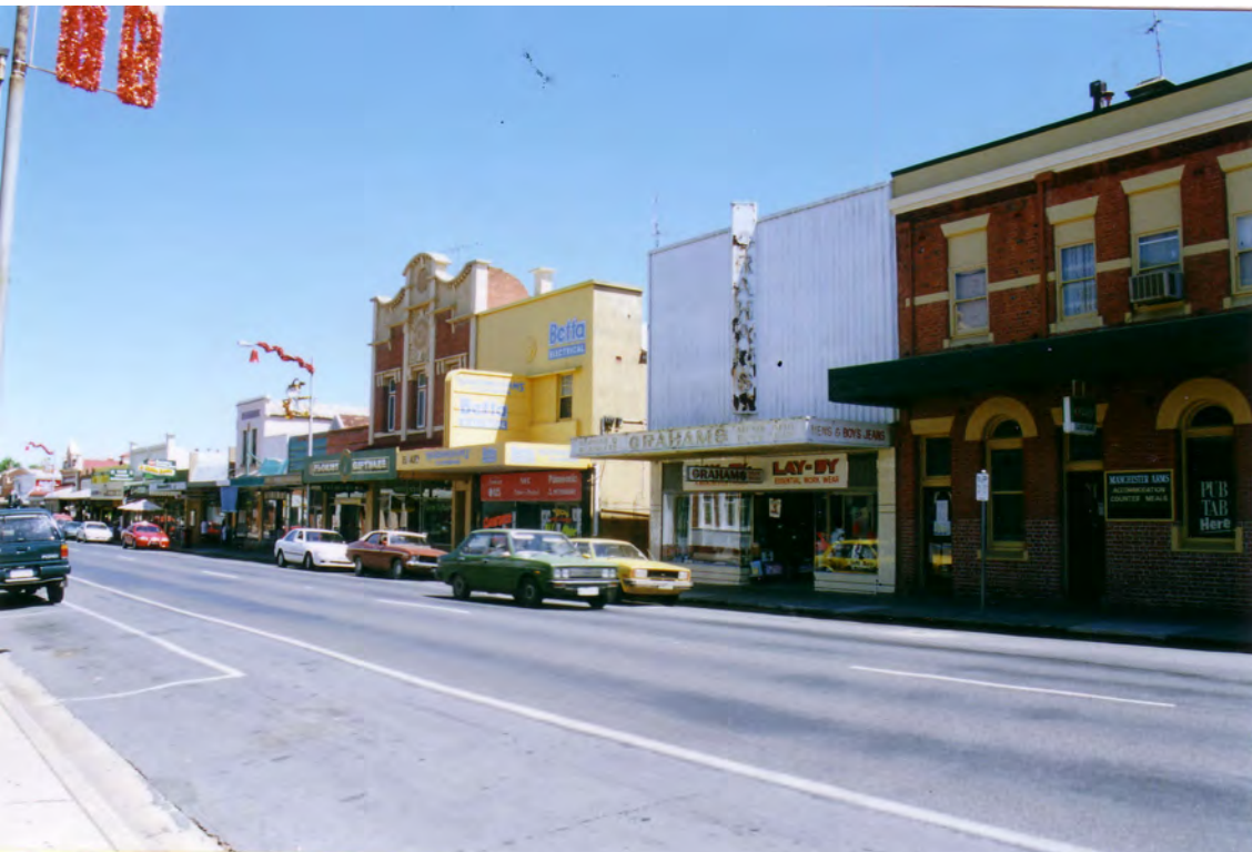
Photo 1.02: Napier Street west side between Alma and Raglan Streets. Note the introduced cantilever verandahs, early dominant parapet of the former St Arnaud mercury building and the shopfronts with ingoos.
