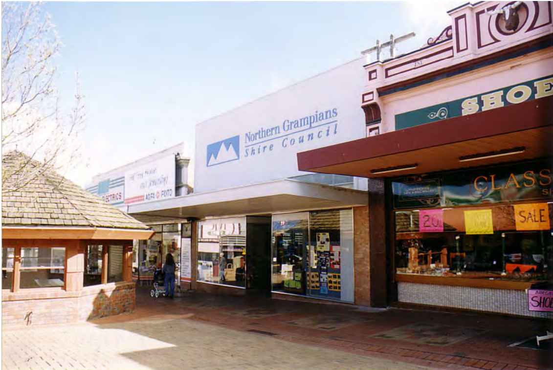
Photo 8.07: Northern Grampians Shire Council shopfront office, showing introduced parapet and shopfront.
