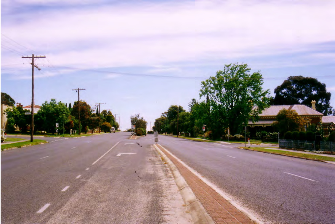
Photo 6.07: Seaby Street, showing the narrow introduced median strip between Luke and Johnson Street.
